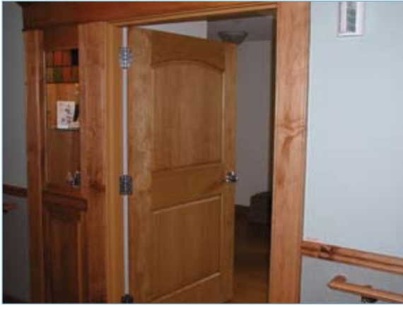
Installed door at Assisi Heights.
