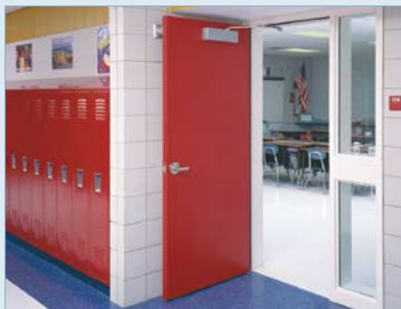
VT door installed in an elementary school.
