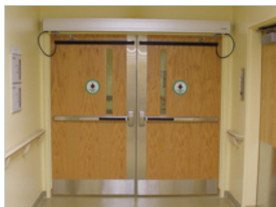
Doors featured an ASSA ABLOY hardware package, Sargent exit devices and mortise locks and Norton closers.
