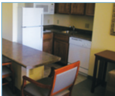
Postformed countertops feature Wilsonart DeepStar Bronze laminate design and Nova edge profile.
